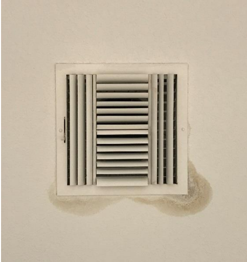
Condensation damage
