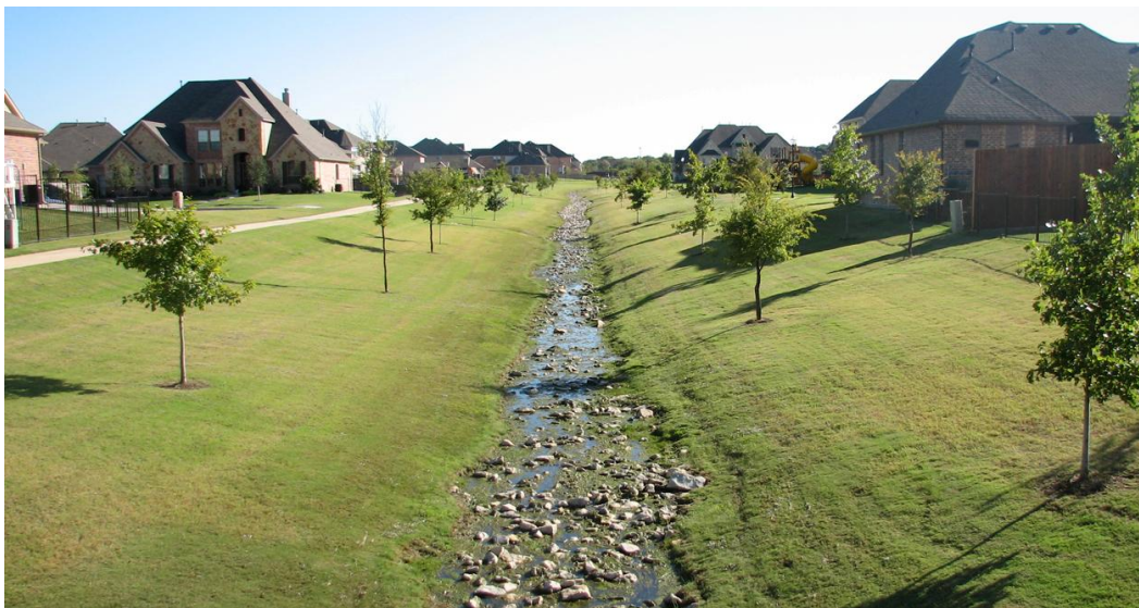
Although this is an attempt to provide visual and physical access to a drainage way, it is unfortunate that the original meanders and creek side vegetation crucial to the viability of the ecosystem were removed.
