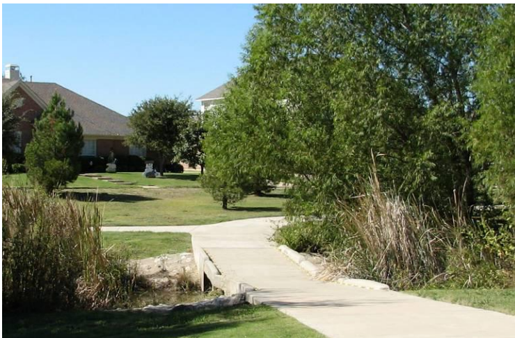
The low water pedestrian crossing at the creek has reflectors on either side which makes it safer at night. Ideally, the width should be increased to 12’ minimum to allow cyclists and other users to pass safely, which is wider than the city’s current standard of 10’ minimum.
