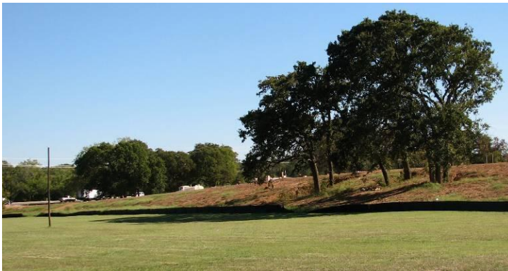
The elevated access roadway puts mature trees at a disadvantage and compromises their life expectancy due to extensive fill within the drip line of the tree.
