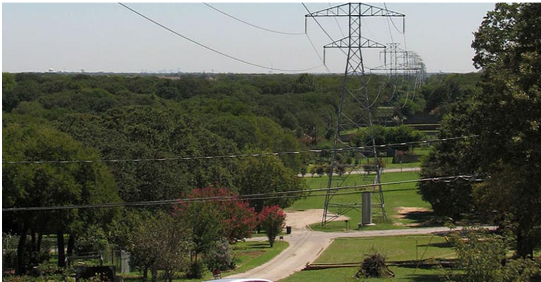
The prominent location of a water tower on a high elevation within the City provides an opportunity to celebrate views to the surrounding landscape.
