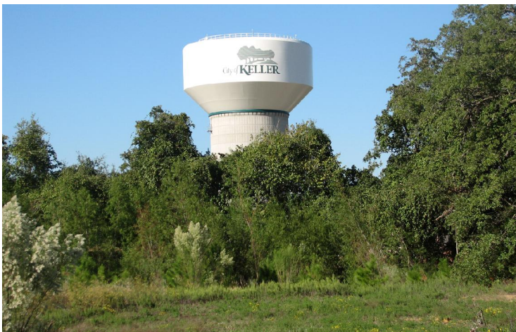
The presence of water towers in Keller is prominent due to their size and visibility from afar.
